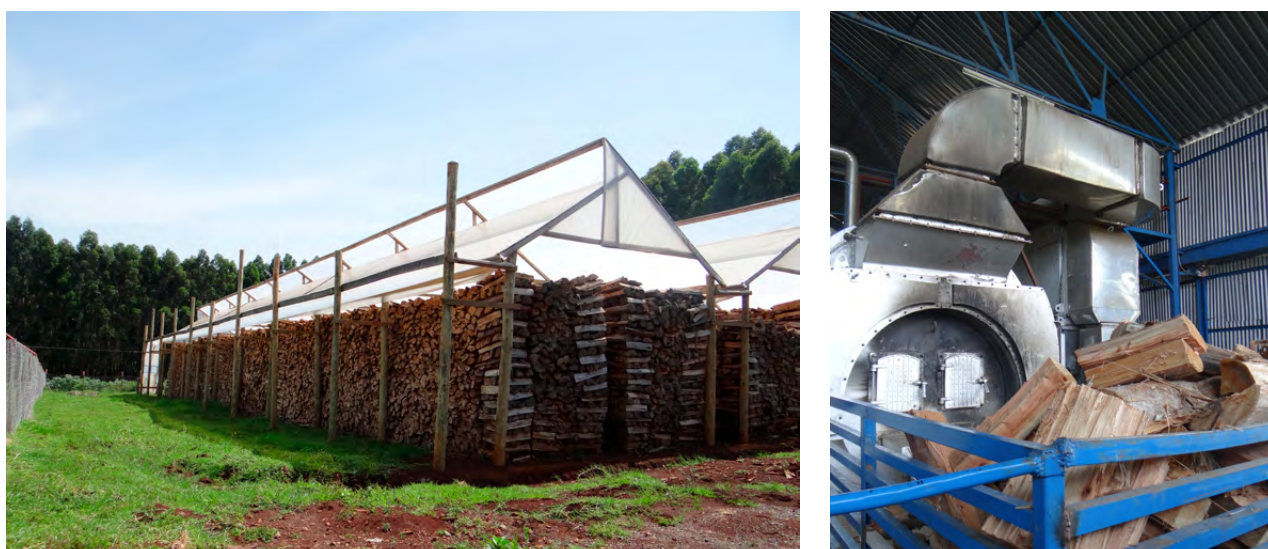
FIGURE 19: Wood drying before use in a boiler fed by woody biomass at Finlays estate (Kericho)
