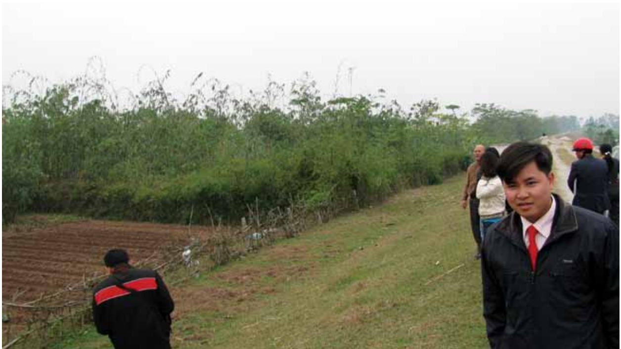
The dense bamboo forest in An Hoa has shown to give effective protection to the river dyke.
