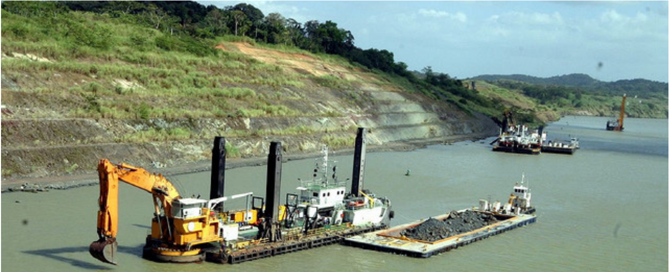
Excess sediment regularly needs to be dredged to ensure proper functioning of the Panama Canal.
