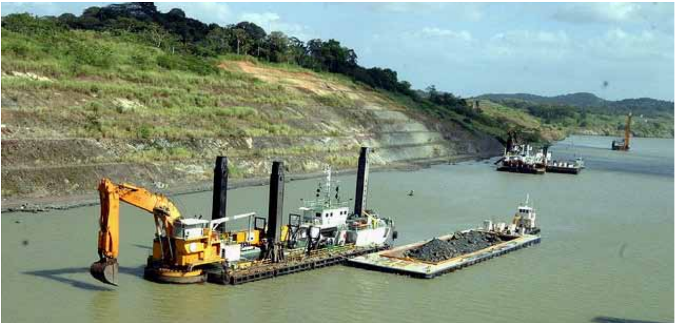
Excess sediment regularly needs to be dredged to ensure proper functioning of the Panama Canal.
