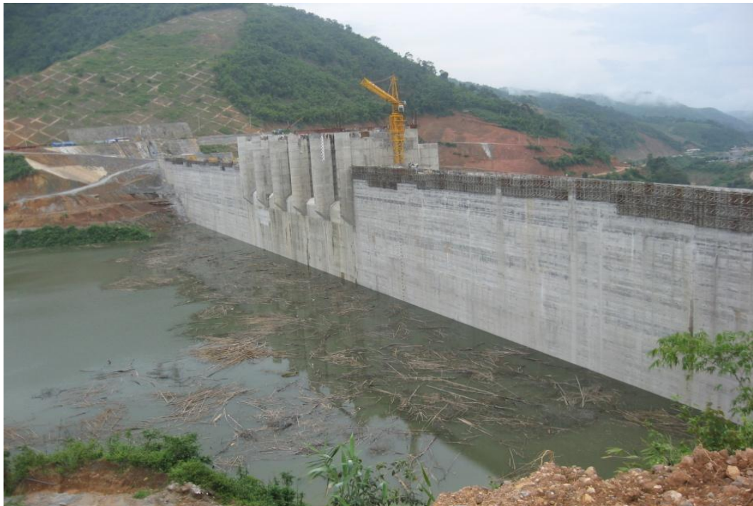
Figure 07: Dong Nai 3 hydro-power
