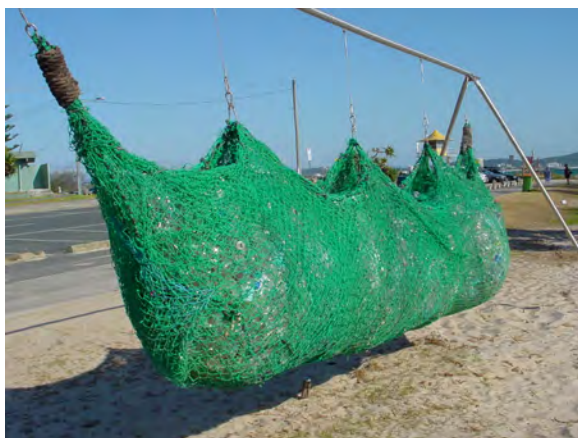
Figure 88: Recycled fish nets full of plastic bottles (left) could be used to provide protection to mangrove seedling planting areas where high wave action prevents seedlings becoming established (e.g right figure).
